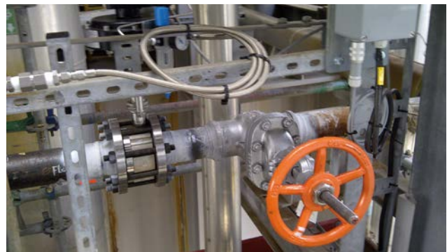
Fig. 6 The new sliding gate valve with 8049 positioner.
